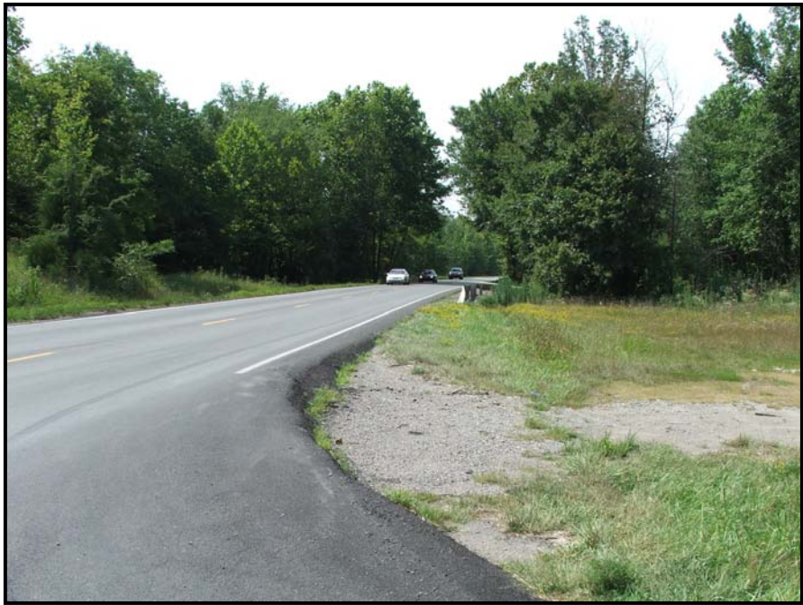
Looking north at US 431 from Cleaton Road, east approach (Location 1-T)
