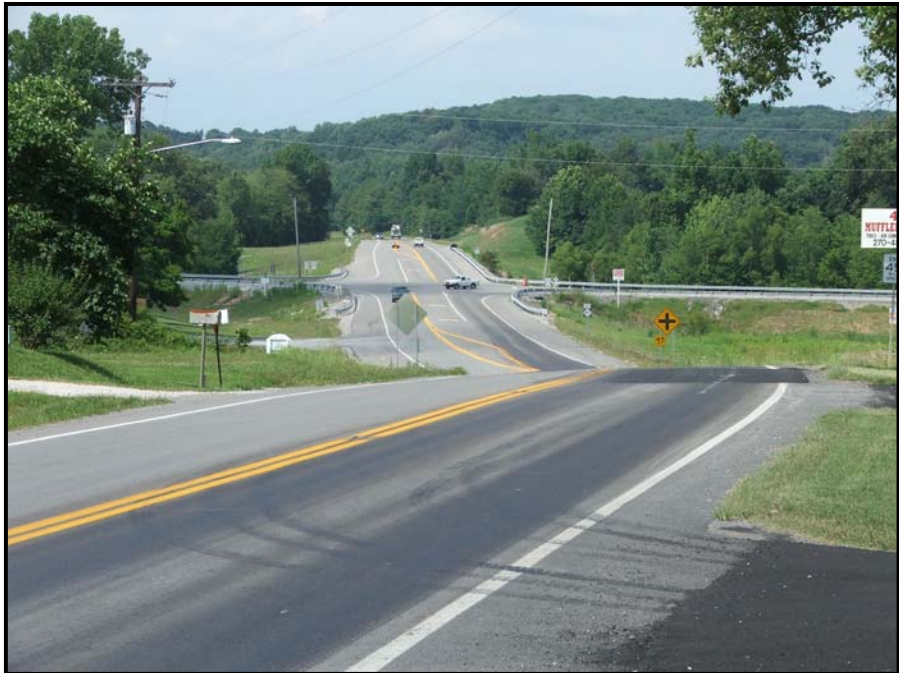
US 431 intersection with KY 85, facing north, seen from crest at Main Street intersection in Island (Location 2-F)
