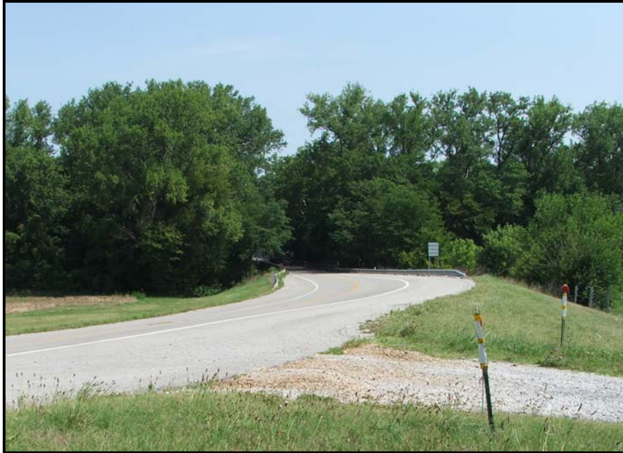
View north towards bridges at Location 1-A
