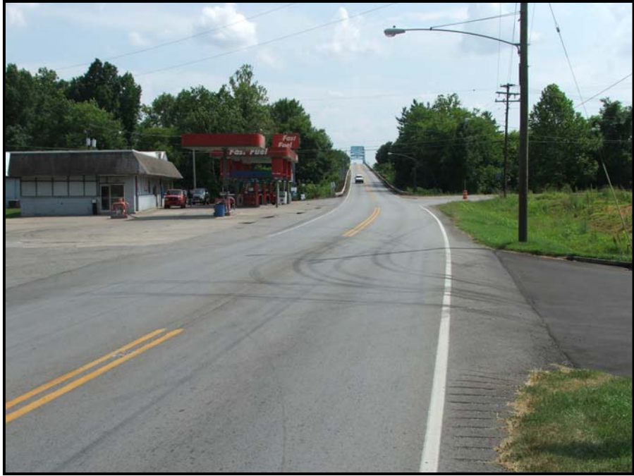
View south towards Green River Bridge and intersection with Third Street in Livermore (Location 2-G)
