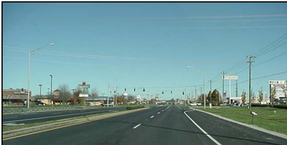
Recently improved four-lane commercial strip in south Owensboro approaching US 60 Bypass at Location 2-O.
