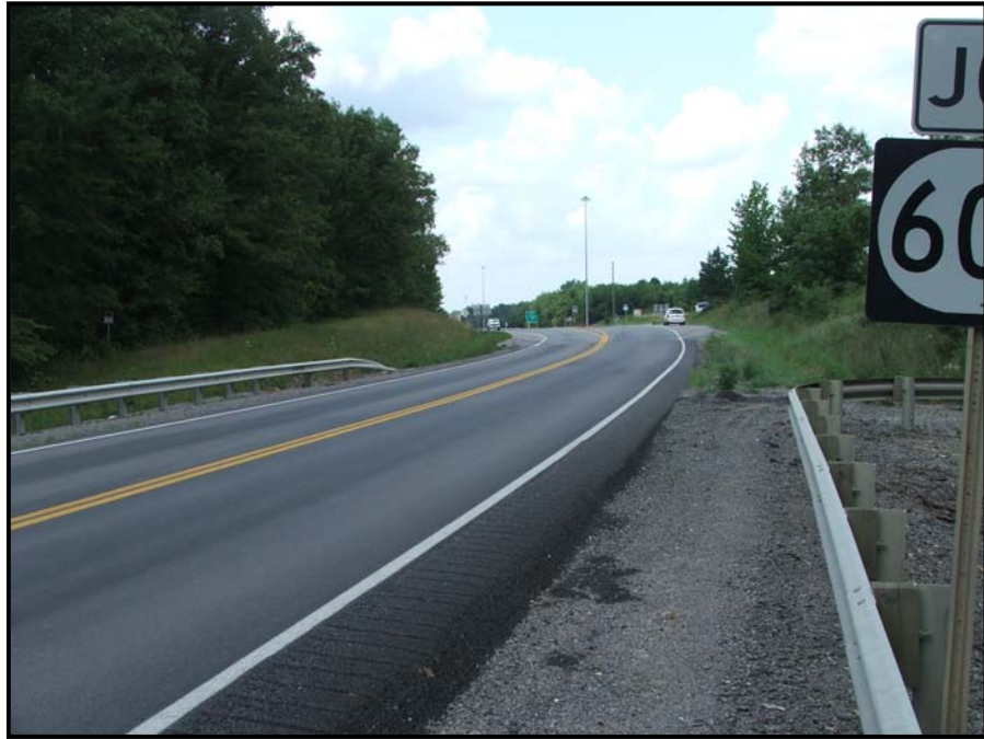
View north towards Western Kentucky Parkway, with transition from two-lane to four-lane section at Location 1-U
