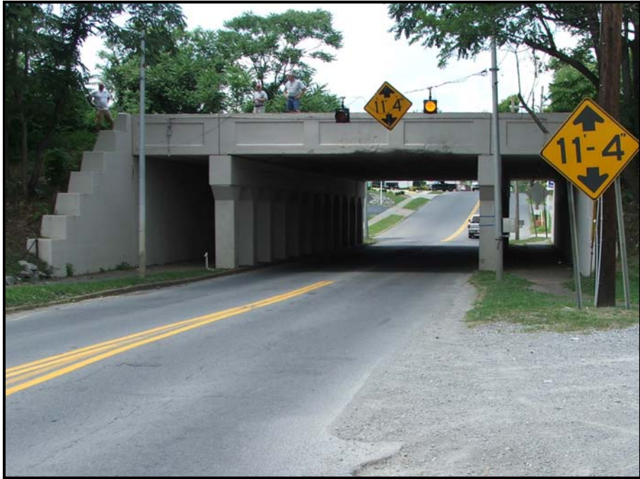
Low railroad overpass in Central City within Location 2-B
