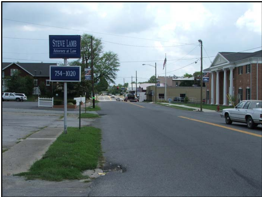
US 431 in Central City, approaching intersection with KY 70 at Location 2-B
